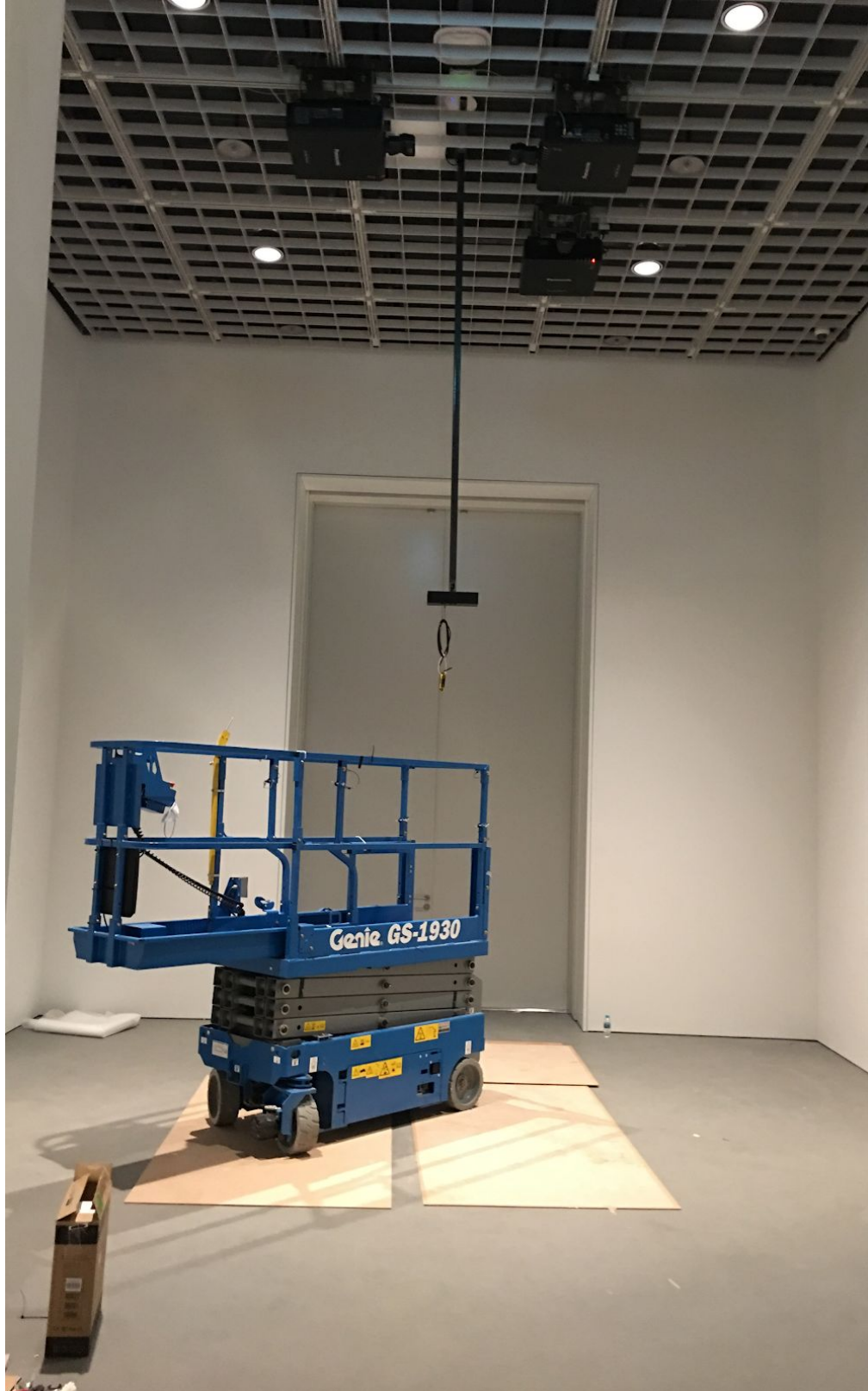
Museum setup: 3 ceiling projectors and a kinect hanging from a square pole.
